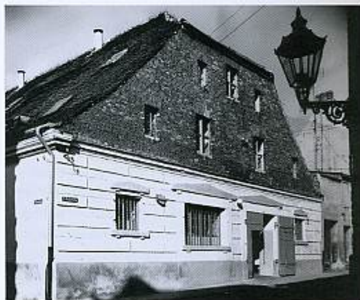
The building of Wozownia before adaptation Photo: Archives of Wozownia Gallery
